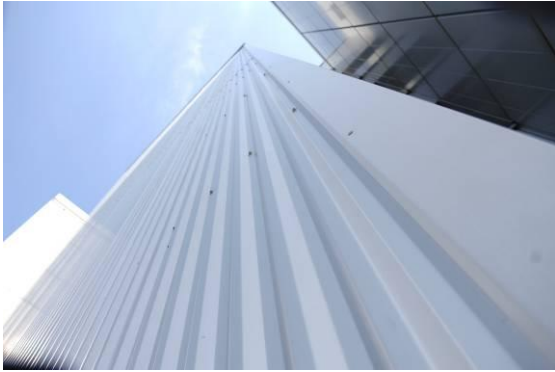
Chrome-free coil coated V-groove sheet performing well after 10 years service, even at its most sensitive point – the dripping edge.
